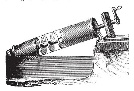
Experiment with your Archimedes screw. How high can you lift water? Raise the upper container, and tilt the screw upward at a steeper angle.
